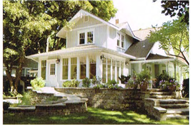
Green and sustainable elements are incorporated into this two-story addition at a historic Walla Walla home.
