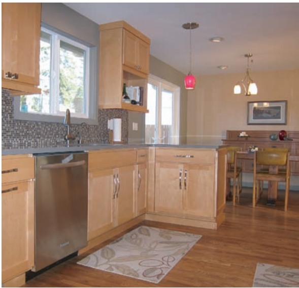
Looking towards where wall was demolished
