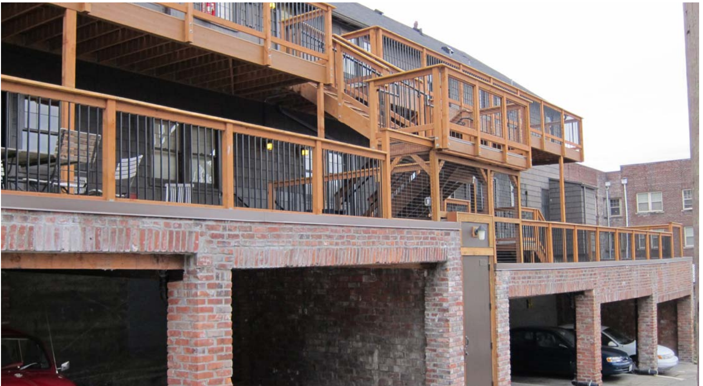
View of New Railings and Parking Garage
