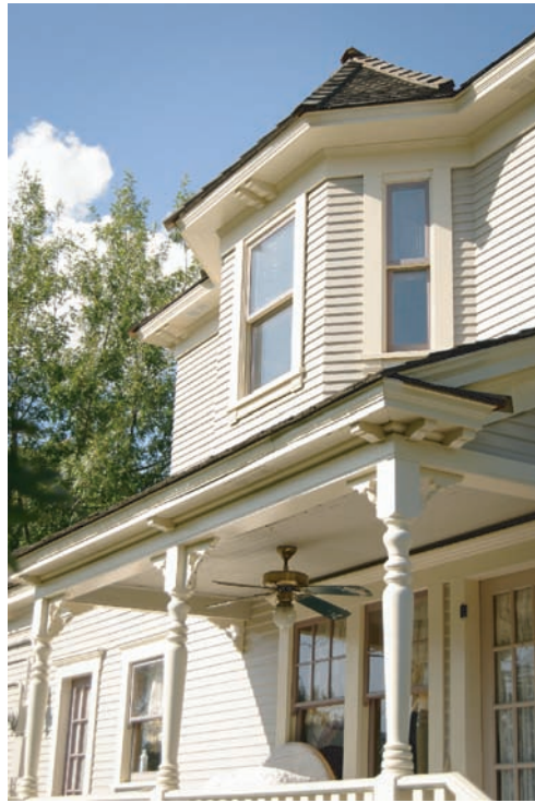
Exterior - The new second story master bathroom blends in with the original structure
